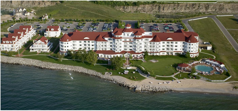
The Inn at Bay Harbor
